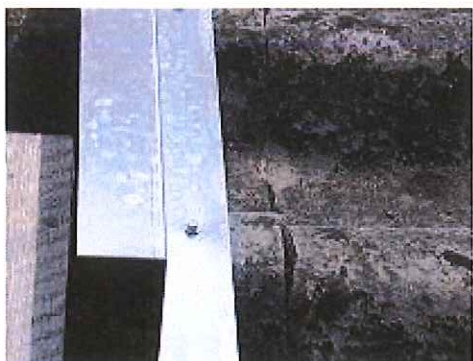
Pictures 3 & 4 Zed spacer fixed through top of sheet corrugation
