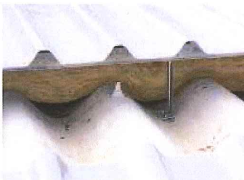
Picture 2 Bar & bracket with sheet and insulation
