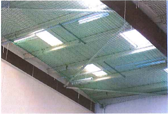
Picture 5 Close hung internal safety nets
