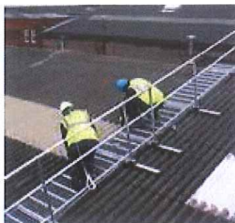
Picture 8 Staging with hand rail and safety line
