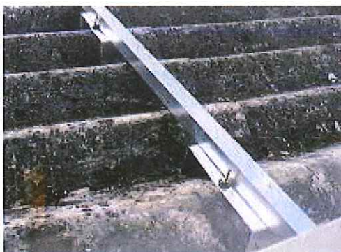
Pictures 3 & 4 Zed spacer fixed through top of sheet corrugation
