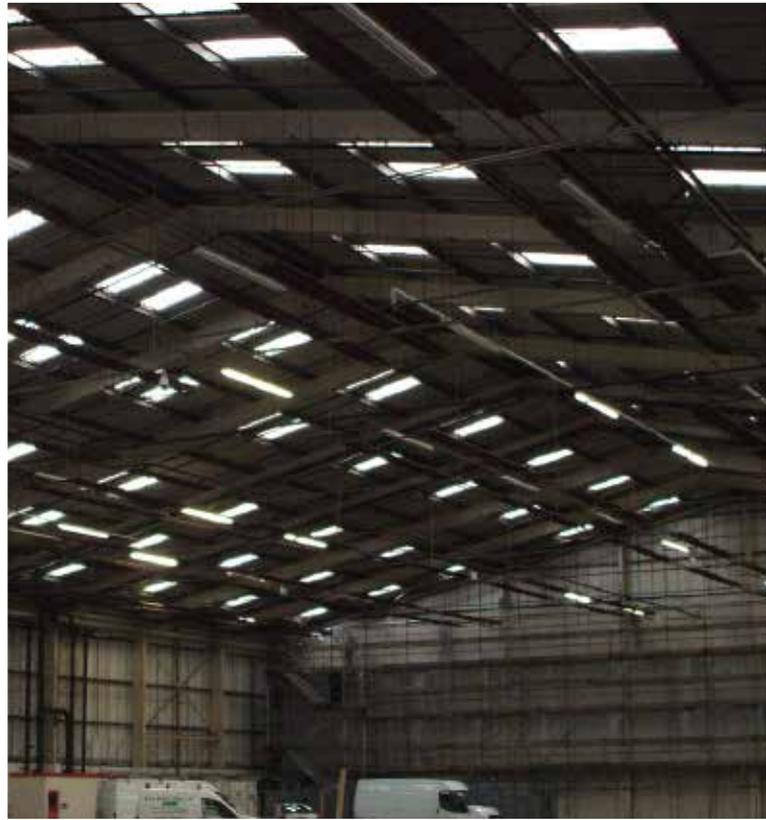
We agreed a Kingspan KS1000RW composite panel and combined with new triple skin rooflights and modern single skin overlay to the side cladding, and now have achieved a modern day, light and attractive building which achieves a huge energy saving and leak free environment.
