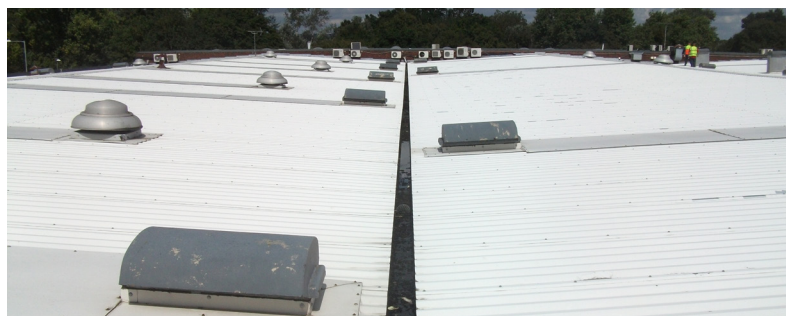
The roof has been over-clad and there is little room to easily access the gutter for cleaning etc
