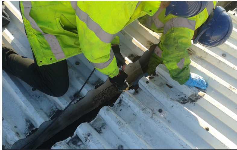
New Unifold gutter system being installed
