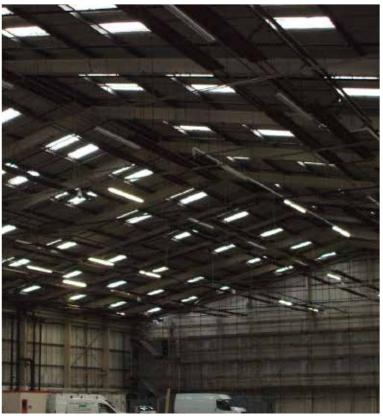
We agreed a Kingspan KS1000RW composite panel and combined with new triple skin rooflights and modern single skin overlay to the side cladding, and now have achieved a modern day, light and attractive building which achieves a huge energy saving and leak free environment.
