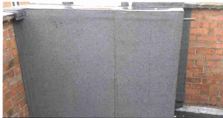
After: Water tank housing rebuilt and refelted
